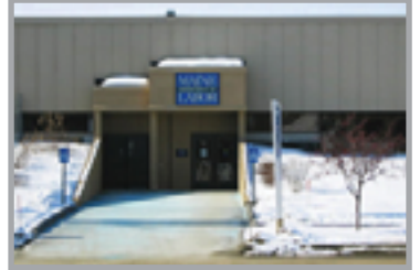
SafetyWorks, Maine Dept. of Labor 45 Commerce St. • Augusta, ME
