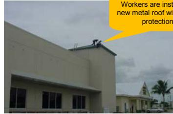
Workers are installing a new metal roof without fall protection.
