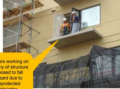
Workers working on balcony of structure exposed to fall hazard due to unprotected side/edge.
