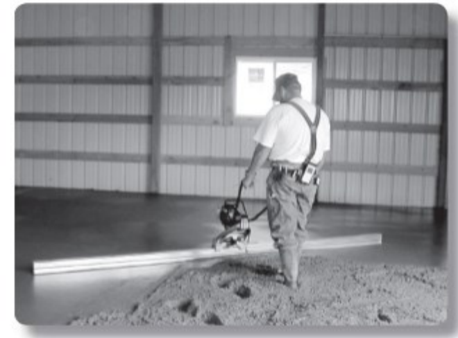
Solution: Motorized screeding
