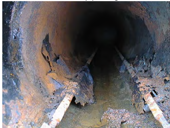
Leaking HCl Cylinder in 5502 ERCV after 1 year
