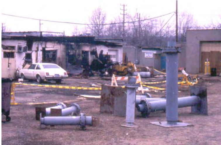
ERCV's Used By NJ DEP after Gollub Explosion 1988
