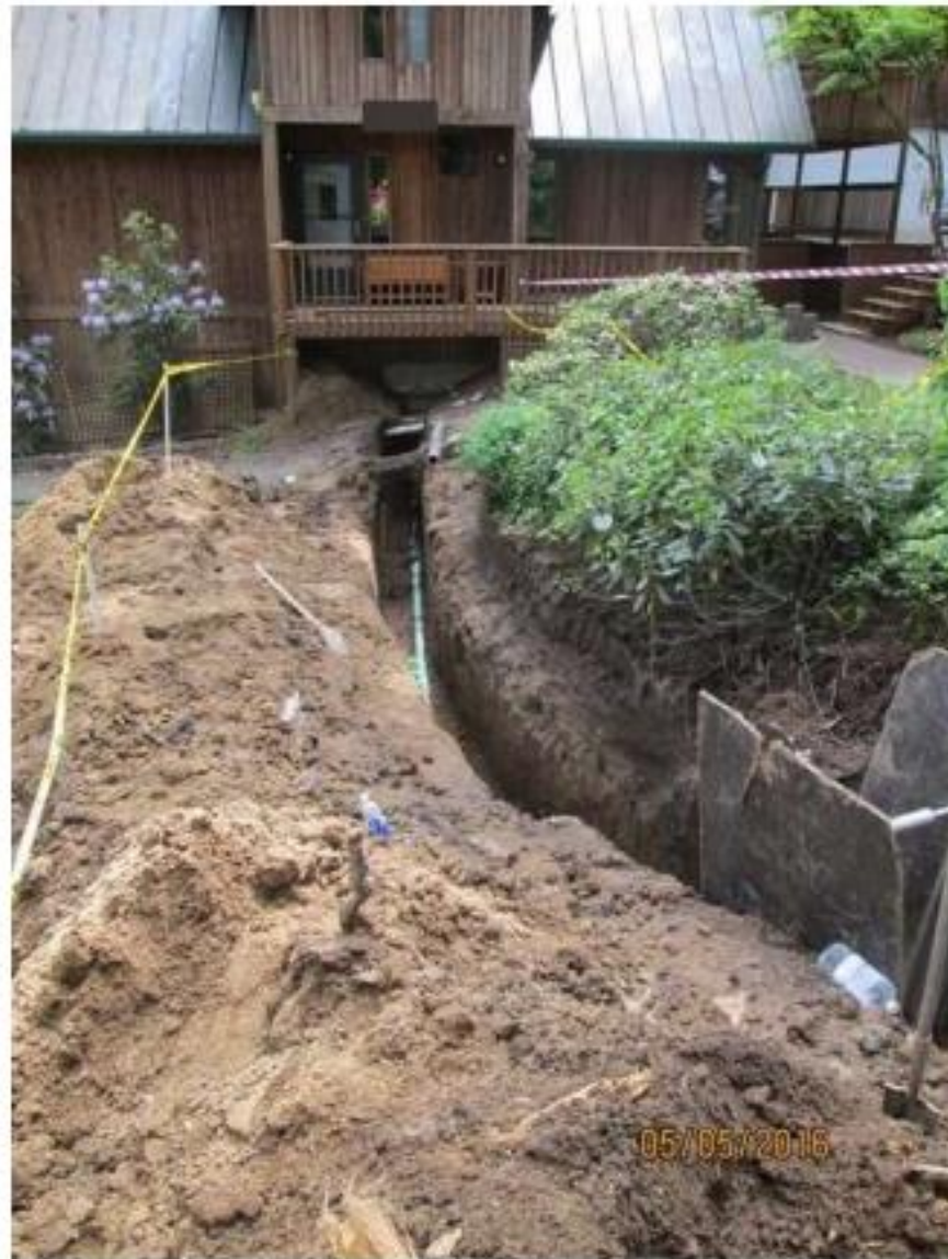
Figure 3. View of trench work area in front of house
