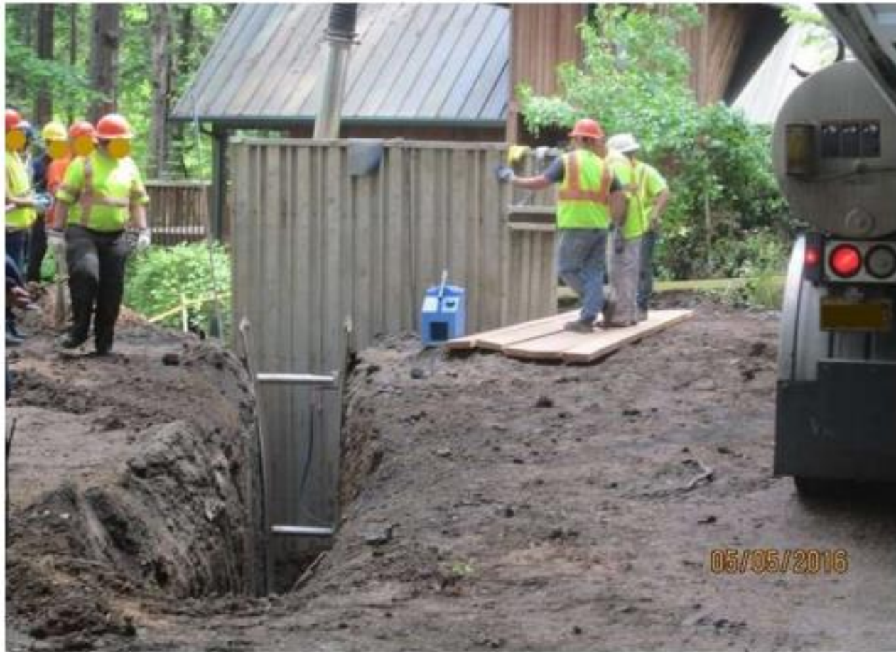
Figure 2. Emergency responders preparing to install a trench box before starting rescue and recovery work, to prevent risk of additional collapse and injuries
