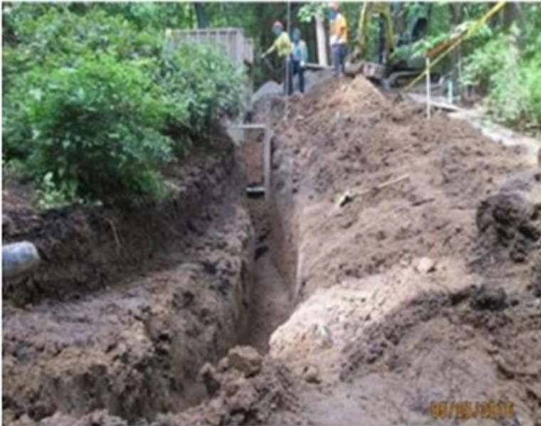
Figure 4. View from house showing trench work area and general soil conditions
